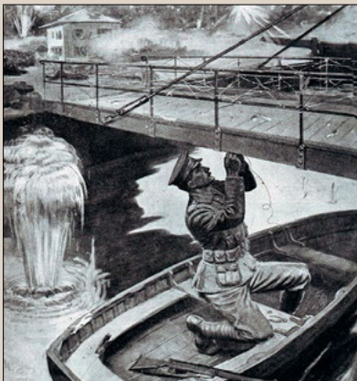
Above: Lance Corporal Charles Jarvis, of 57th Field Company Royal Engineers, preparing the demolition of the bridge at Jemappes, Mons, for which he received the Victoria Cross
