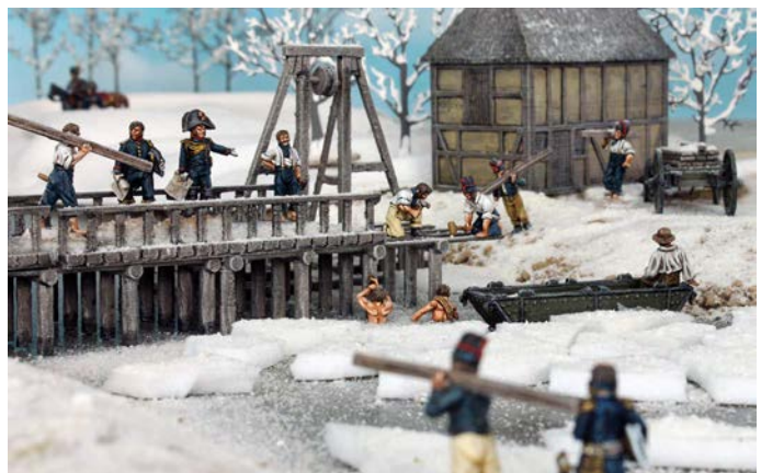
Above: Jouselin, inspector of the Ponts et Chaussées, supervises the repair of the bridge (Perry Miniatures).
