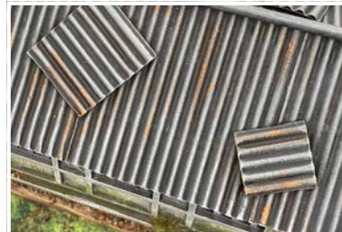
Above: Sheets of corrugated card, painted with a simple metallic drybrush then weathered with rust make for realistic warehouse roof sections.
