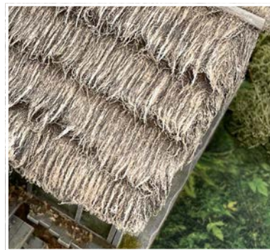
Above: Thatched textures add a touch of remoteness to some of the buildings, making them more suited to the jungle location.
